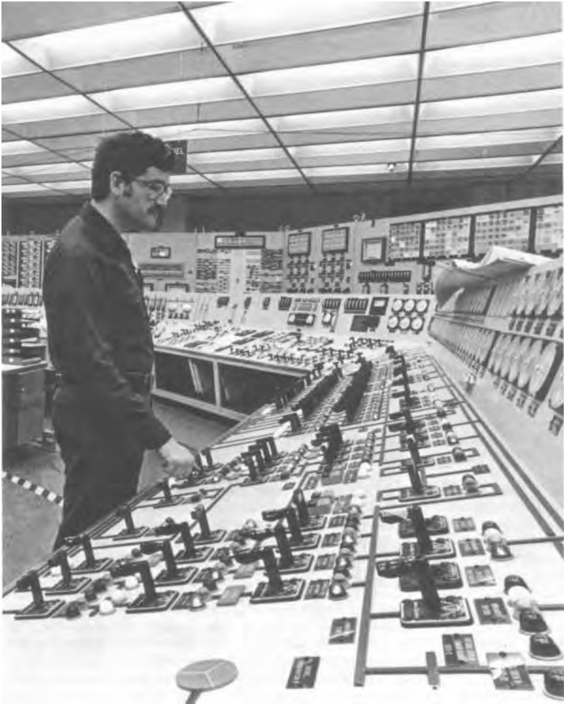
The size and layout of the Unit 2 control room may have contributed to the operators' difficulties in responding to the accident.
